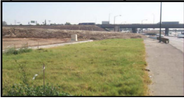
Figure 5-2 Grassed Buffer Strips
