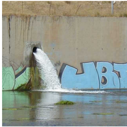
Glendale LA Water Treatment Plant Effluent Outfall
