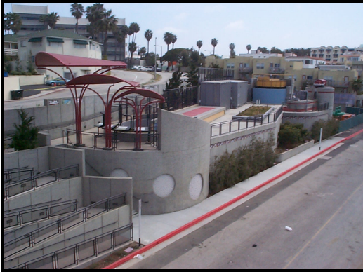
Figure 5-10 Santa Monica Urban Runoff Recycling Facility (SMURRF)
