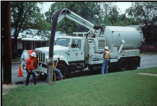
Figure 5-17 Catch Basin cleaning
